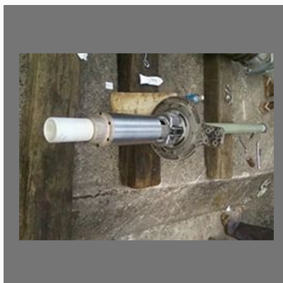
Circuit Breaker Overhauling
