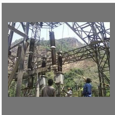
Circuit Breaker Overhauling
