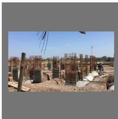
Foundation Construction Service
