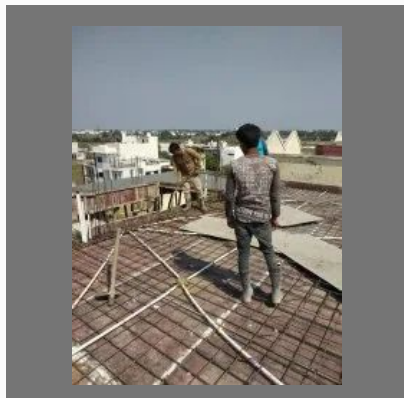
Slab Casting Work
