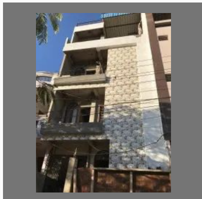
Civil Renovation Work
