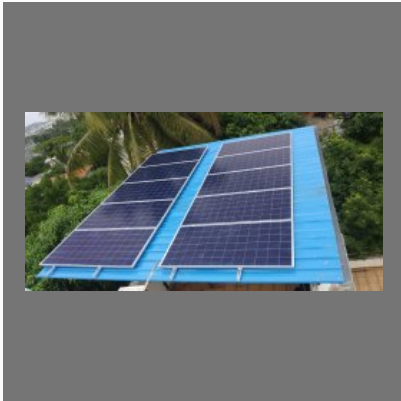
Rooftop Solar Panel Structure
