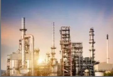
Essential Oil Processing Unit Setup
