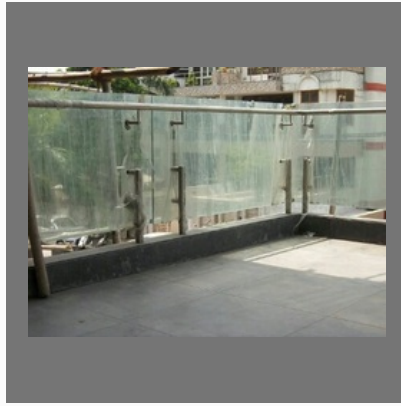
Front Glass Railing
