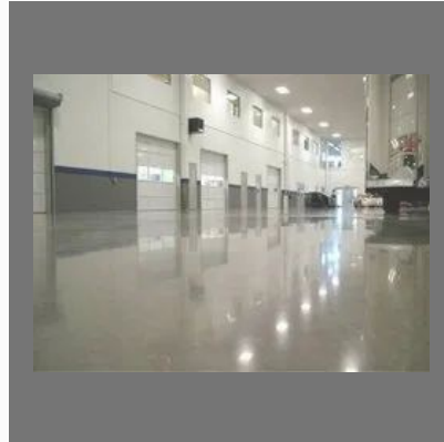
Water Based Epoxy Coating
