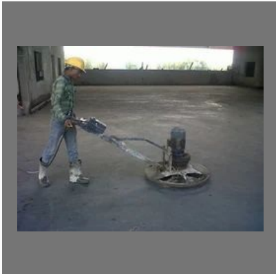
VDF Flooring ( Trimix Flooring)
