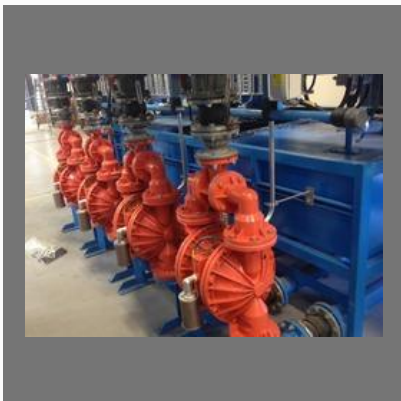
Wilden Pump Maintenance
