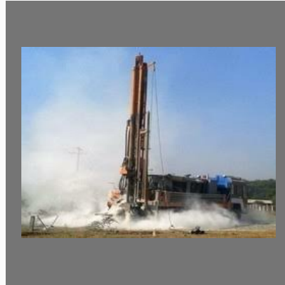
New Borewell Drilling
