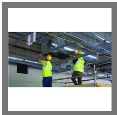
Ventilation System Installation Service
