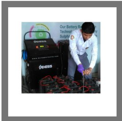
Battery Life Extension
