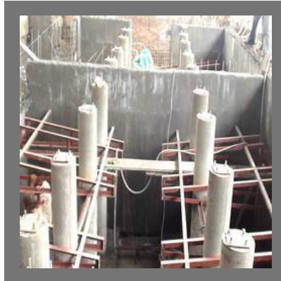
Paint Booth Foundation (Wet & Dry)
