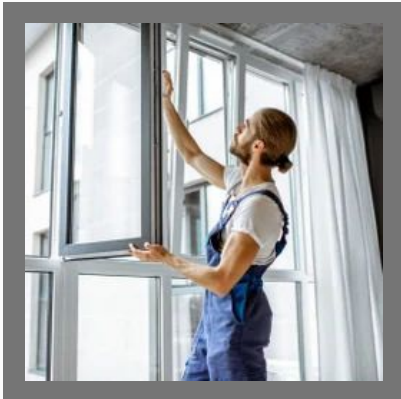
Aluminium Window Repairing Service
