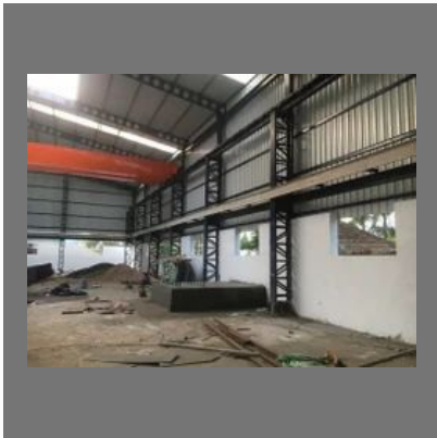
Shed Fabrication Contractor
