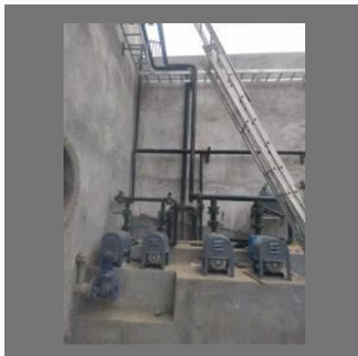
Industrial Piping Installation Service
