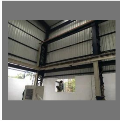
Platform Fabrication Works
