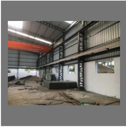
Industrial Shed Fabrication
