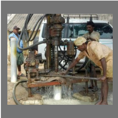
Drilling Contractors Services
