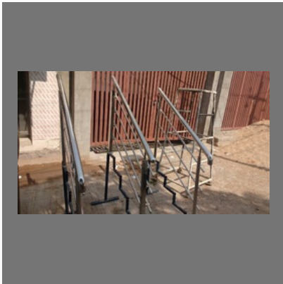
Steel Staircase Railing
