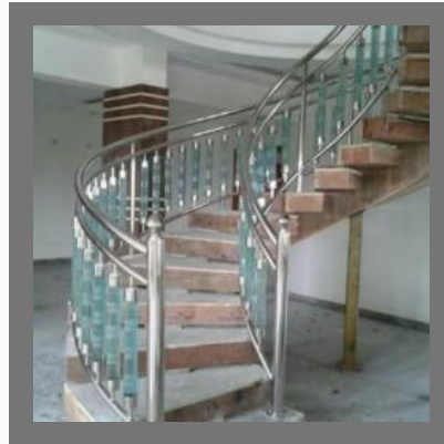
Stainless Steel Hand Rail Fabrication
