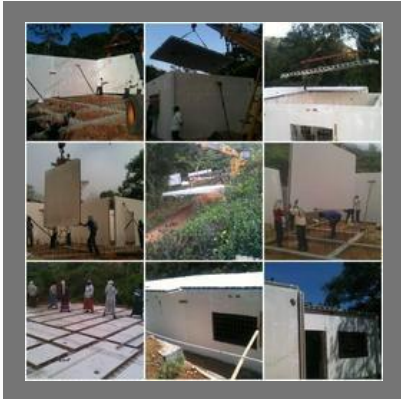
GFRG Residential Construction
