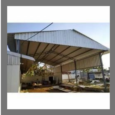
Commercial Prefabricated Structure
