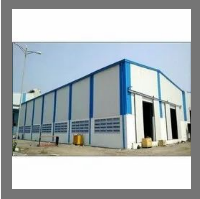
SS Prefabricated Building Structure
