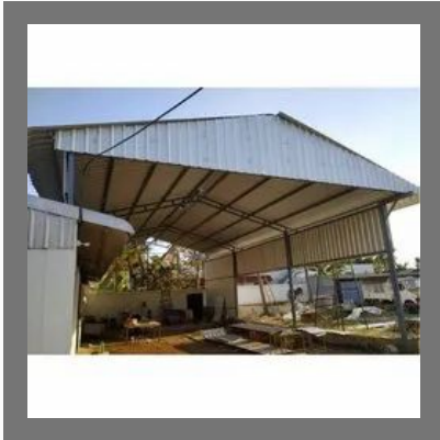
Factory Roofing Shed
