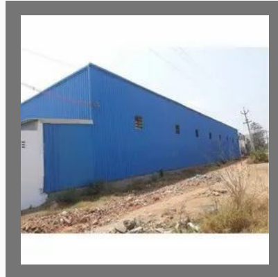
Industrial Prefabricated Shed
