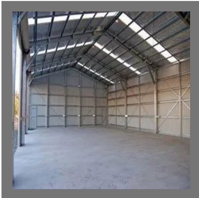
Steel Prefabricated Shed
