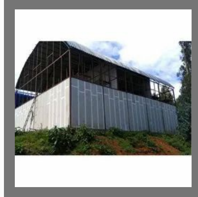
Pre Engineered Industrial Building Structure
