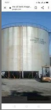
MS Oil Storage Tank
