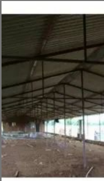
15 Mm Industrial Shed
