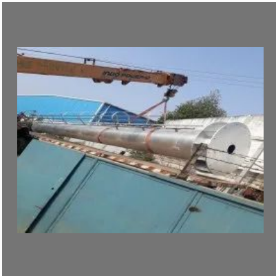
Industrial Mild Steel Chimney
