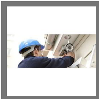
CCTV Camera Repair & Installation Services
