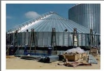
Structural Erection Services
