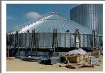
Equipment Erection Services
