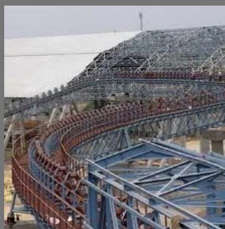
Structural Steel Erection Services
