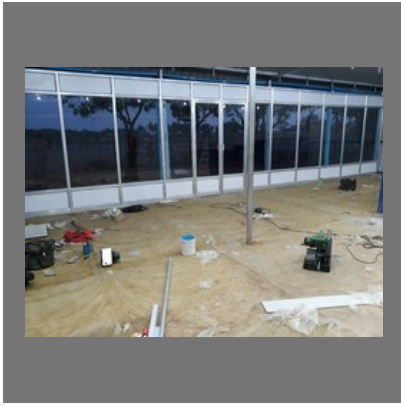
All Aluminium Partition & Window Work
