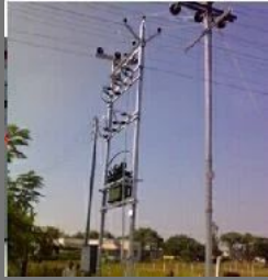
Schools Electrical Works
