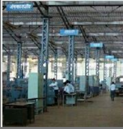
Offices Electrical Works
