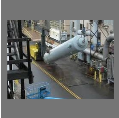
Rigging & Equipment Service
