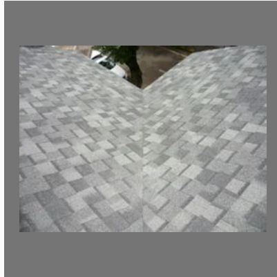
Gray Roofing Shingles
