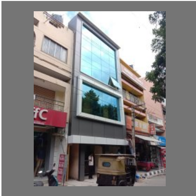
Acp And Glass Glazing
