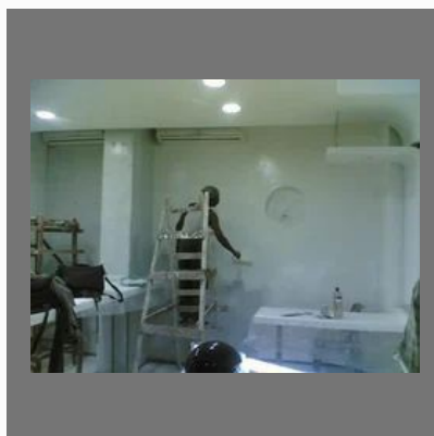
Epoxy Coating Service
