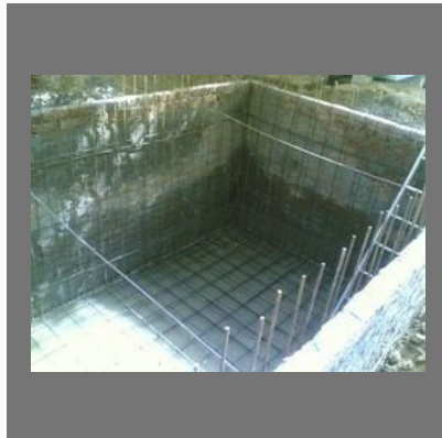
UG Sump Waterproofing
