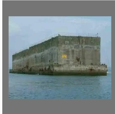
Watertight Structure Repairing Service
