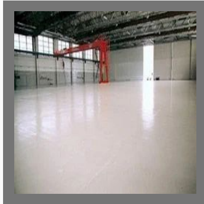
Epoxy Underlay Screed
