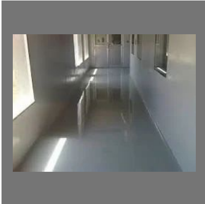
Polyurethane Coating Service
