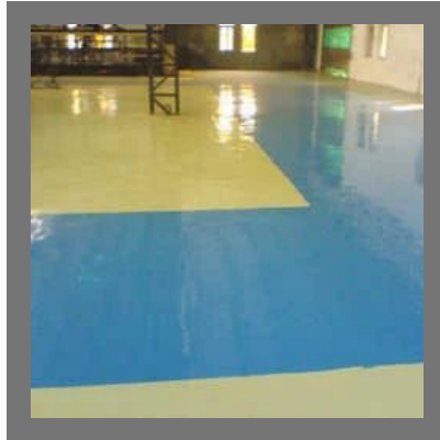
Self Leveling Epoxy Flooring
