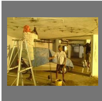
Pressure Injection Grouting Service
