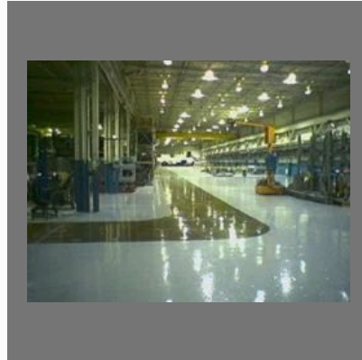
Epoxy Flooring Service
