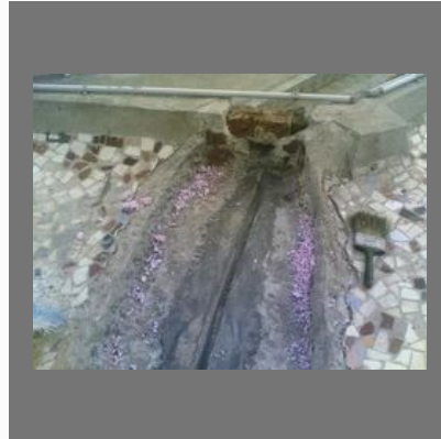
Expansion Joint Treatment Service
