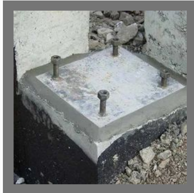
Foundation Grouting Service
