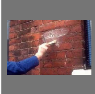
Brick Wall Waterproofing
