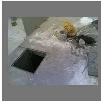
Overhead Tank Waterproofing
