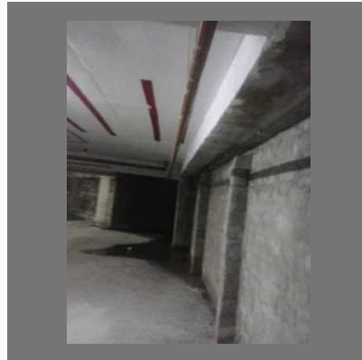
Construction Joint Repairing
