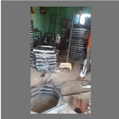
Mild Steel stand Fabrication works
