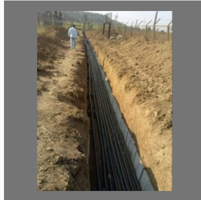
Underground LT Cable Laying Works For Industrial
