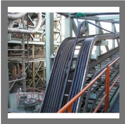
Cable laying Service
