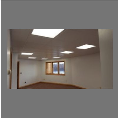
Commercial Wiring Services
