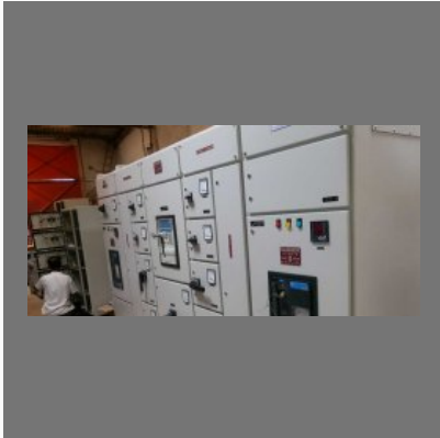
Lt Panels Erection Cable Services
