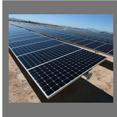
Solar Panel Erection Work And Services
