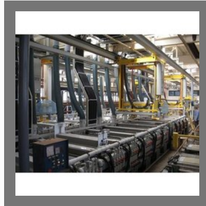
Automatic Nickel Chrome Plating Plant
