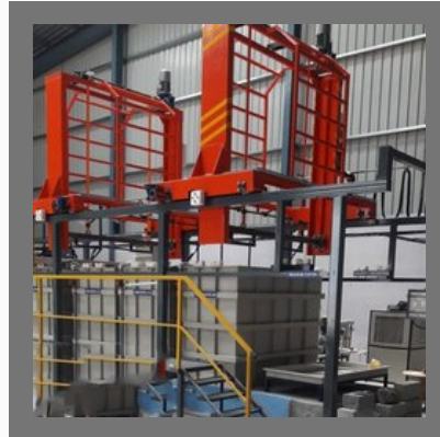
Tin Electroplating Plant
