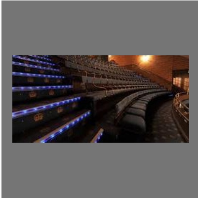
LED Lighting System
