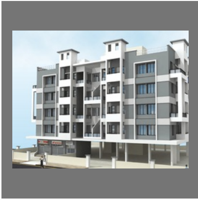
Residential Apartments Construction Service
