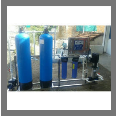
Industrial RO Plant
