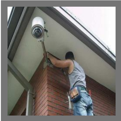
CCTV Camera Installation Service
