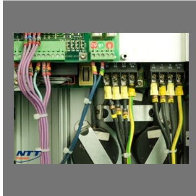
Cable Installation Service/ Training
