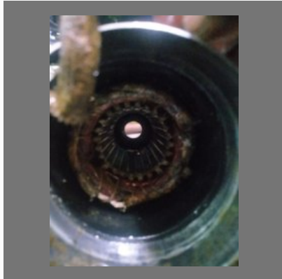
Water Motor Repairing
