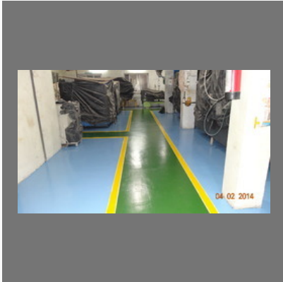
Industrial Flooring Services
