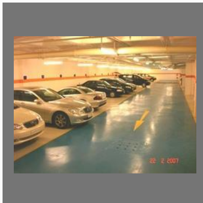
Epoxy Floor Coating Services
