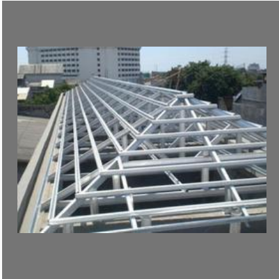
Mild Steel Roofing Structure
