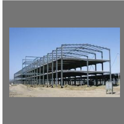
Building Roofing Structure
