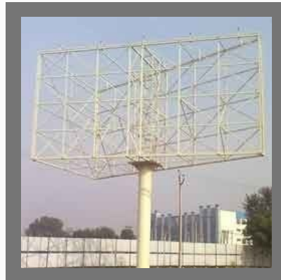
Hoarding Roofing Structure
