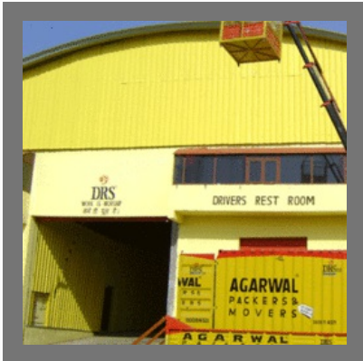
Bulk Storage Facility
