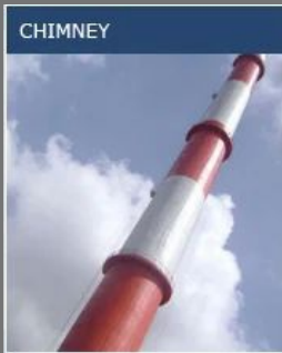
Chimney Constructions Services
