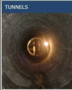
Tunnels Constructions Services
