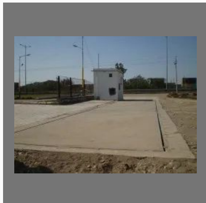
CONCRETE PLATFORM WEIGHBRIDGE
