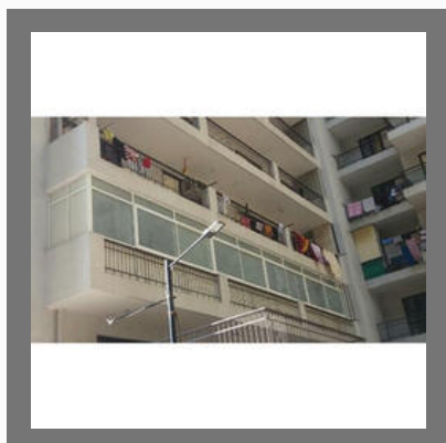
Steel Balcony Railings
