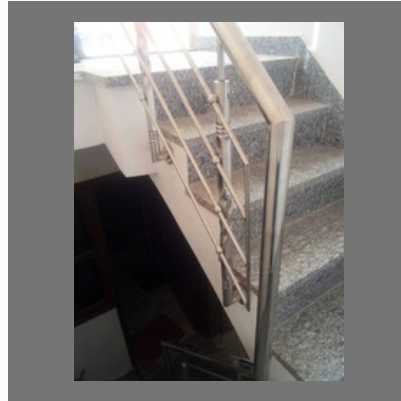
Steel Stair Railing
