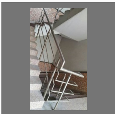
Steel Stair Railing
