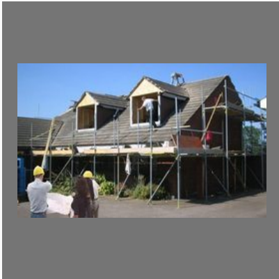
House Construction Services
