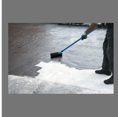
Water Proofing Services
