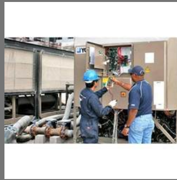
Chillers Repairing Service
