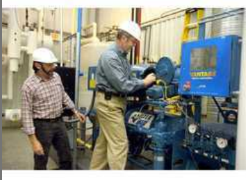
Refrigeration Repairing Service
