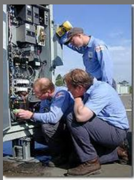
Refrigeration Installation Service
