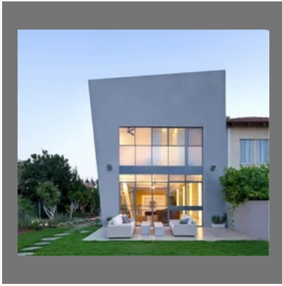
Designing And Executing Special Construction Projects
