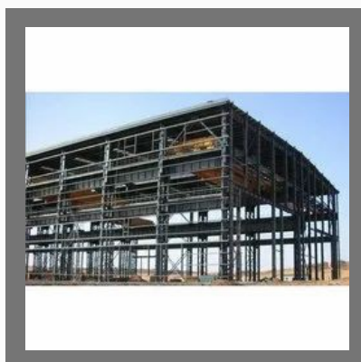
Commercial Building Contractors
