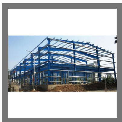
Pre Structural Building
