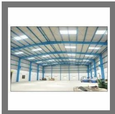
Prefabricated Building Steel Structure
