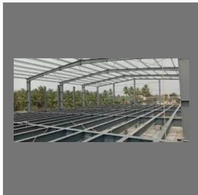
Pre Engineered Building Construction
