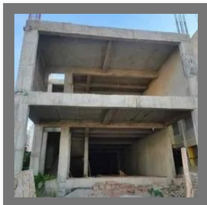
Commercial Building Construction
