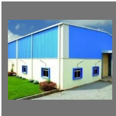
Industrial Building Construction
