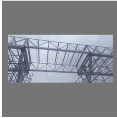
Industrial Structural Fabrication
