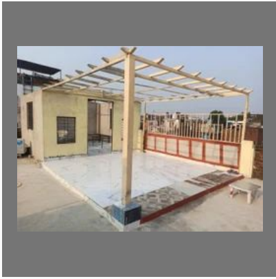
Roof Fabrication Services
