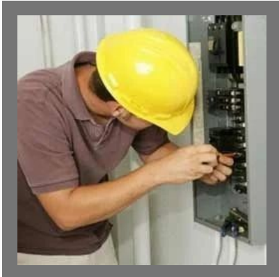
Hospital Electrical Maintenance
