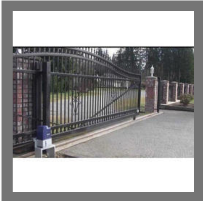
Automatic Sliding Main Gate
