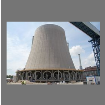
Natural Draught Cooling Tower
